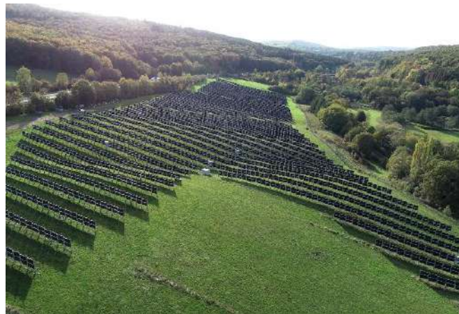
Solar plant in Eppelborn Germany
