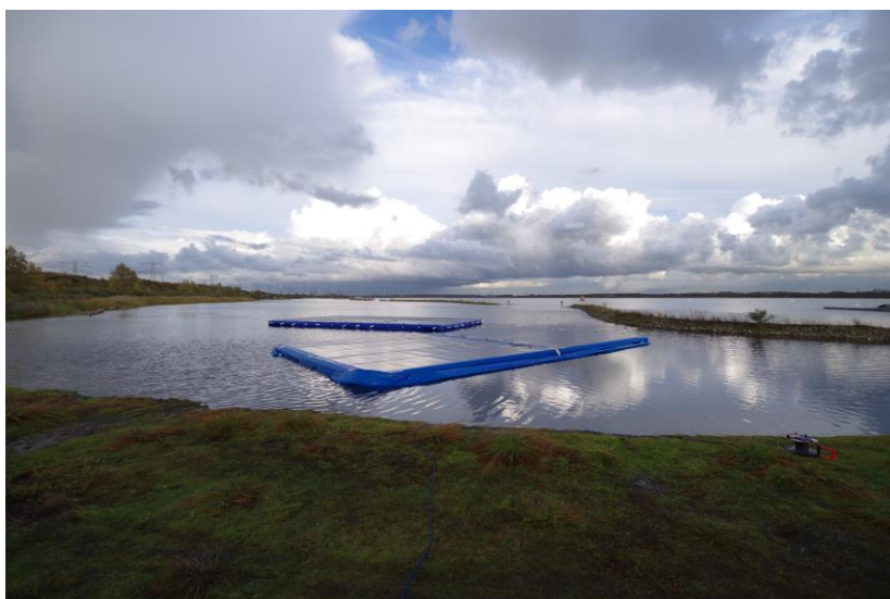
Figure 7: 20 kWp demo system of the Bluewater consortium in the Oostvoornse Meer
