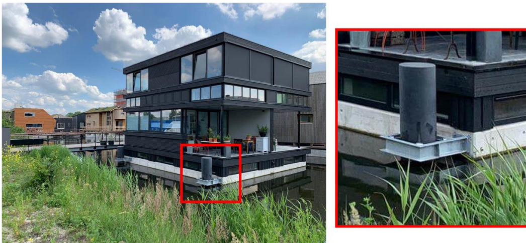
Figure 19 Example of a spudpile solution applied for floating house
