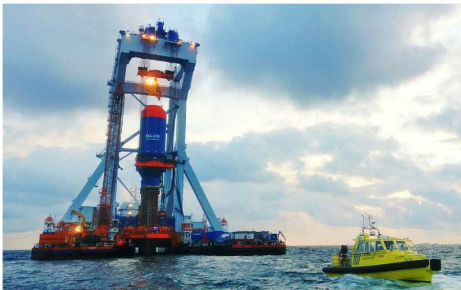
Figure 45 BLUE piling under test (source: IQIP).
