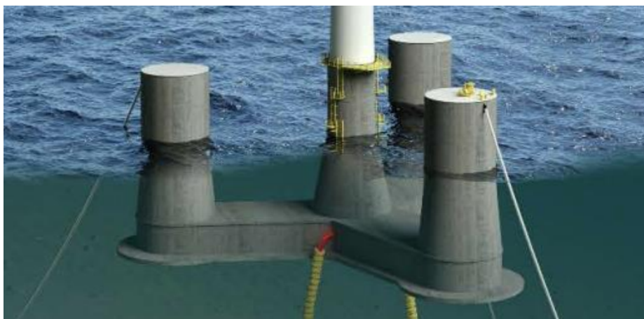
Figure 23 The OO-star semi-submersible concrete floating foundation designed for the Flagship project (source: Flagship project).
