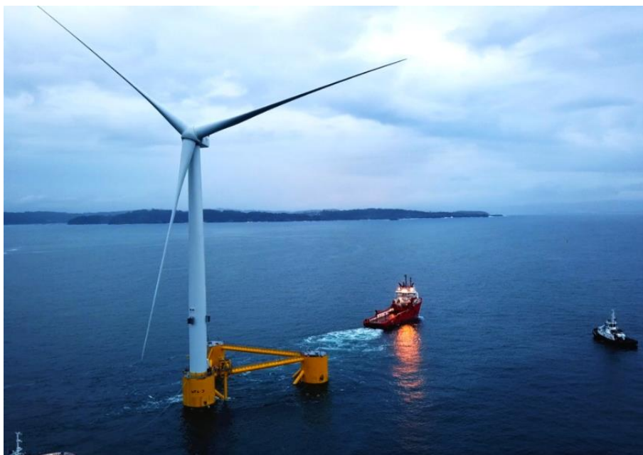
Figure 21 Principal Power's WindFloat semi-submersible and MHI Vestas V164-8.4 MW turbine under tow, Portugal (source: ewind.es).
