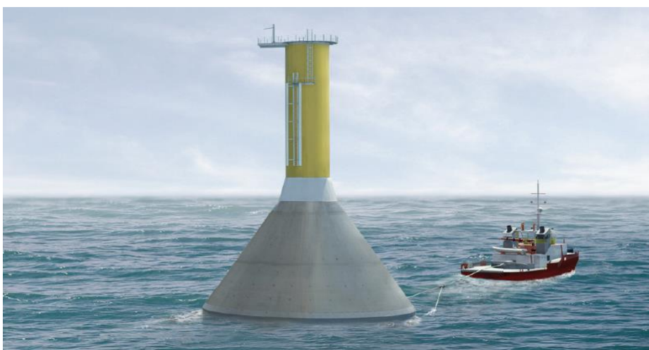
Figure 19 Arup/Costain/Hochtief's Gravitas self-floating GBF (source: Arup).
