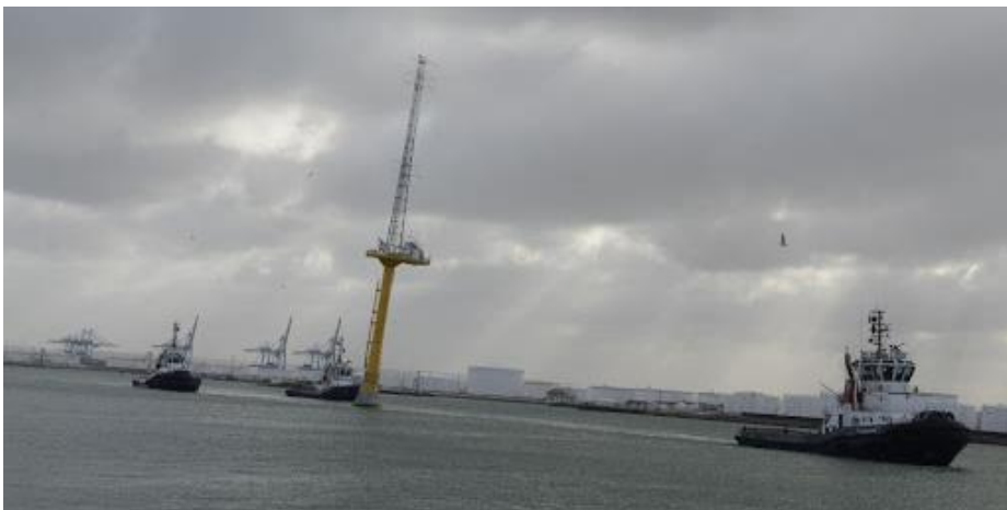
Figure 18 Seatower's self-floating GBF being towed with an offshore met mast to its installation at Fécamp (source: Seatower).
