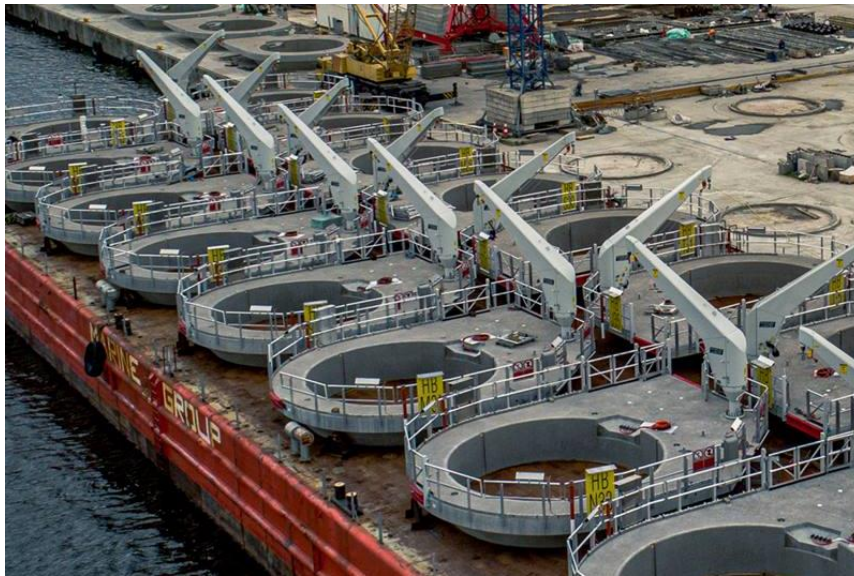
Figure 7 Concrete work platforms (source: Aarsleff).
