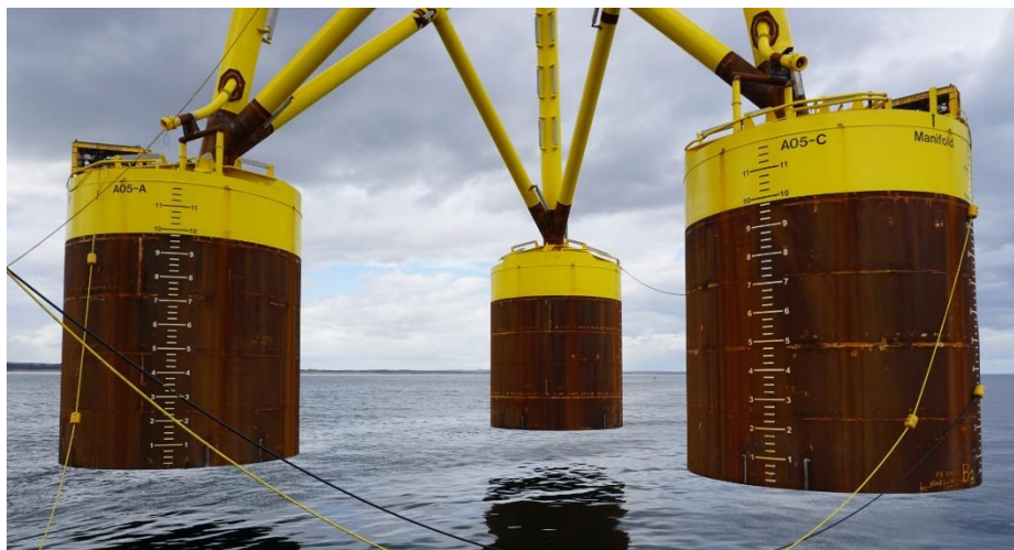
Figure 14 Jacket with suction anchors being installed at Borkum Riffgrund (source: Framo).
