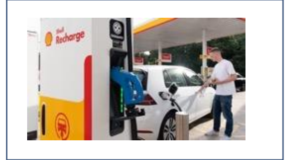
'Ultra' fast charger (>150 kW DC)
