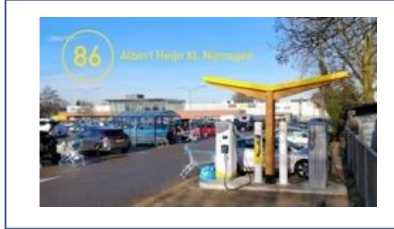
Normale fast charger ( 50 kW DC)
