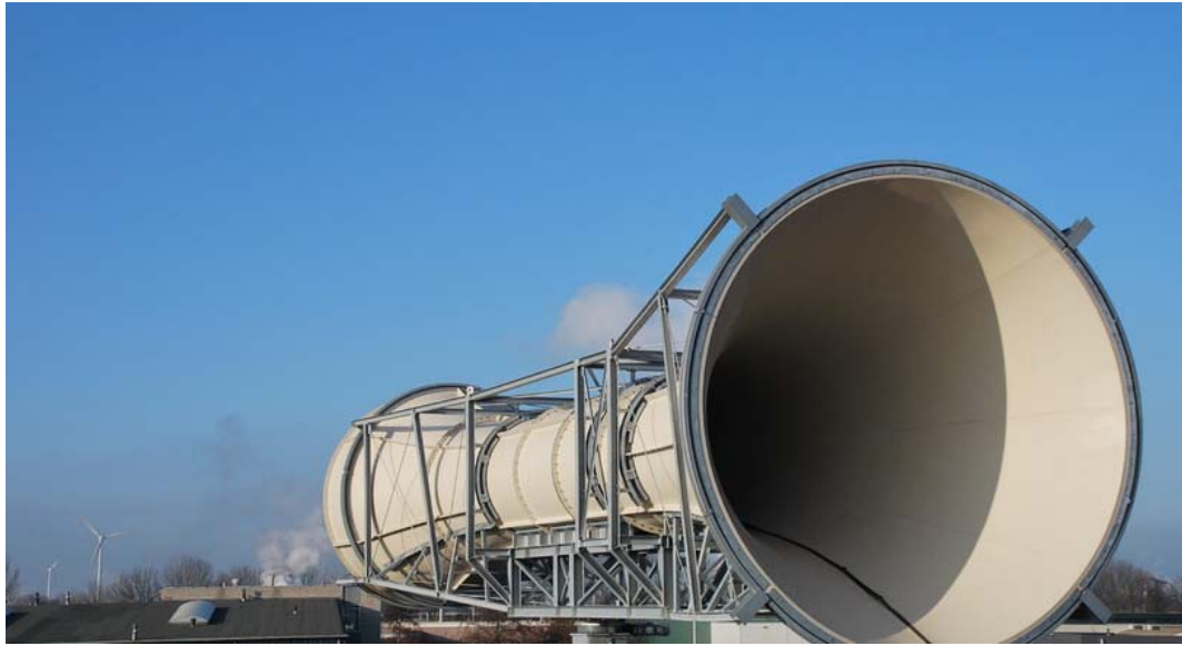
Figure 28. Invelox wind energy system in a straight channel. ( https://www.deingenieur.nl/artikel/proef-met-windtoeter )
