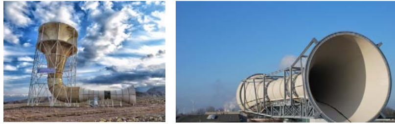
Figure 8. Left: Invelox wind energy system in curved channel. ( https://financialtribune.com/articles/energy/45861/iran-to-employ-efficient-invelox-wind-turbines ). Right: Invelox wind energy system in a straight channel. ( https://www.deingenieur.nl/artikel/proef-met-windtoeter )
