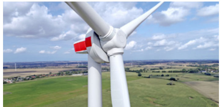
HYGRO specialises in the production, delivery and distribution of hydrogen produced directly from wind. It is building a 4-MW wind turbine with an integrated electrolyser in the province of North Holland. The aim is to maximise synergy between wind power, hydrogen and pipeline & storage technology. The concept optimises conversion of wind power to hydrogen, which can be transported at much lower cost than electricity and with a significantly lower impact on spatial planning.
