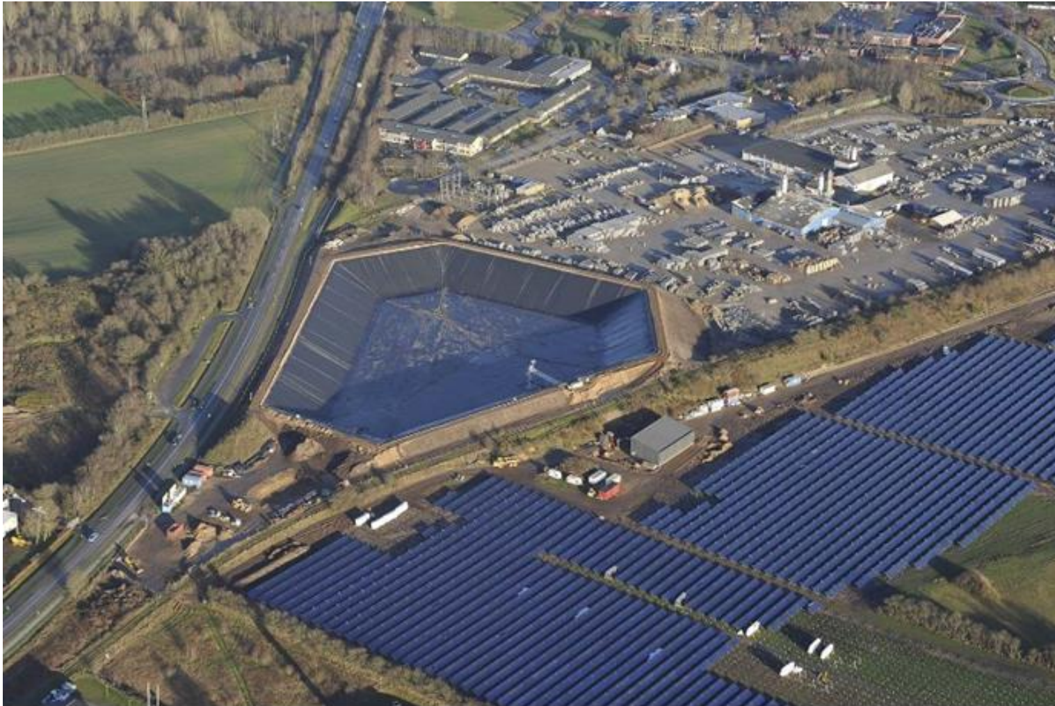
Pit thermal energy storage in Vojens, Denmark. Volume 200.000 m 3
