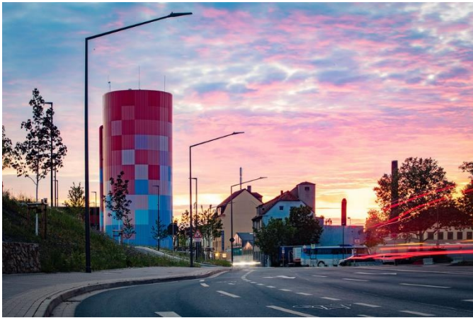
TTES from Stadtwerke Detmold, 1'850 m 3 of water
