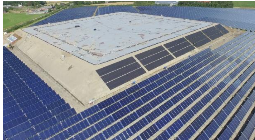
PTES from Gram district heating, 122'000 m 3 of water
