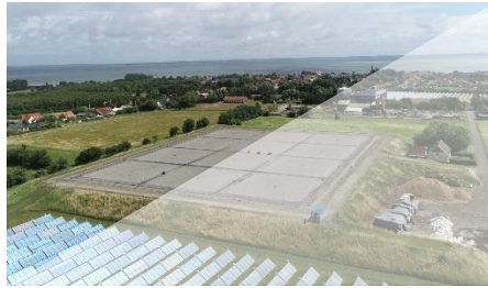
Thermal Energy Storage
