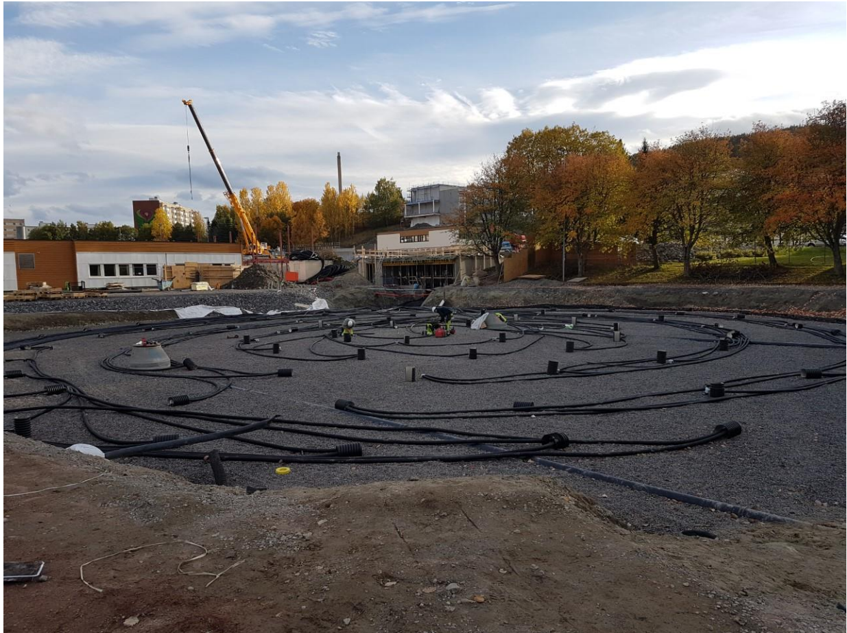
Figure 2: Building site of BTES system at the municipality of Drammen, Norway
